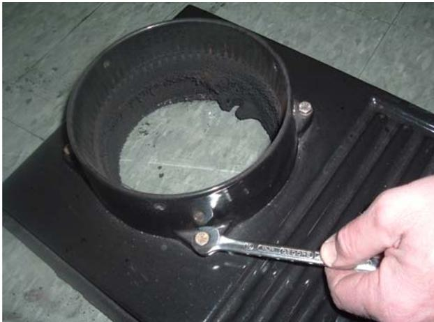
Figure 1: Unbolting the flue collar
