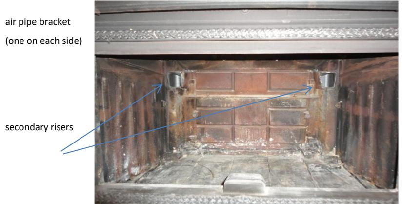
8. To set the air pipe assembly into place, hold the assembly towards the inside front of the stove. Lift the back up, sliding it backwards, pushing it into place. Be sure to tighten the support bolts.
