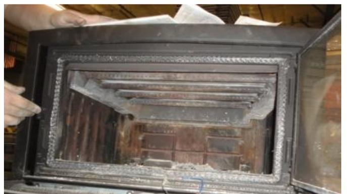
9. Once the air pipe assembly is in place, the bricks can be positioned back into place; Screw the brackets back over the tops of the bricks to secure them.
