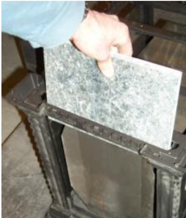
Figure 1- Inserting the Side Stones
