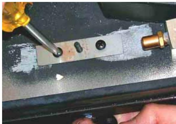
**Photo #6** –Upper plate installed inside the firebox
