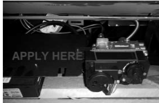
Figure 20 – Valve Warning Label Location
