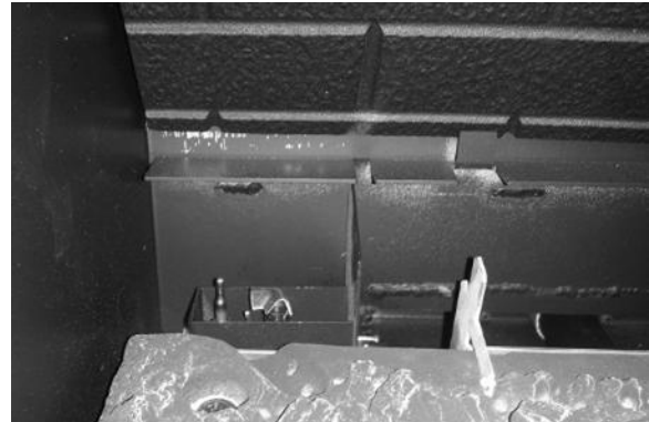
Figure 3 – Pilot, Shield, and Burner Position
