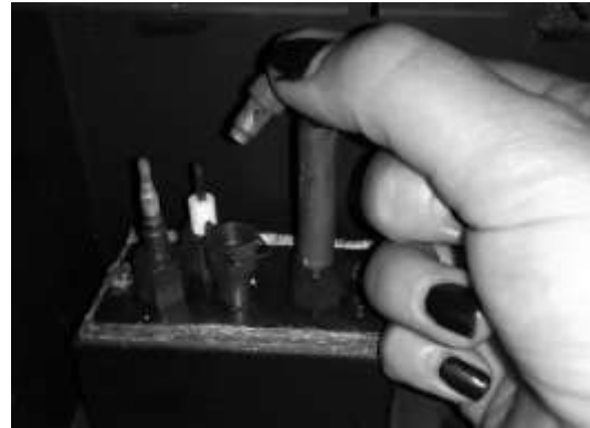
Figure 9 – Replacing Pilot Orifice
