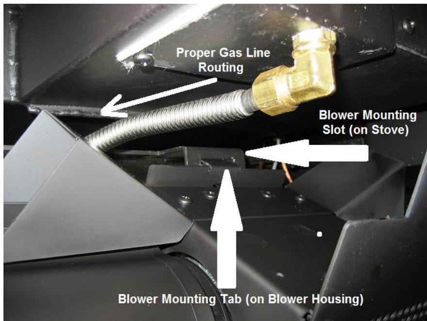
Photo #4 – Blower Tab Inserted in Mounting Slot
