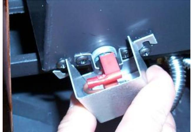
Photo #6 – Snap Switch Protective Cover Installation
