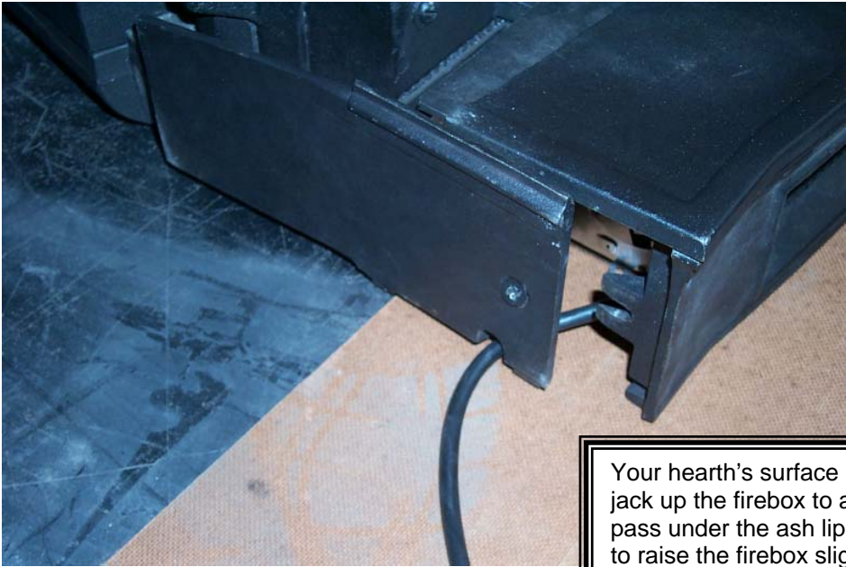
Photo #7 Pass the power cord through the notch in the side casting still mounted to the firebox before pushing the ash lip fully back onto the stove.
